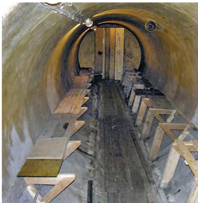
Inside one of the shelters in 2008 before the entrance was filled with rubble
